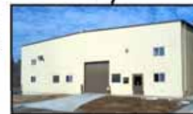
East Annex: Cold Regions Lab and Environmental Flow Facility
