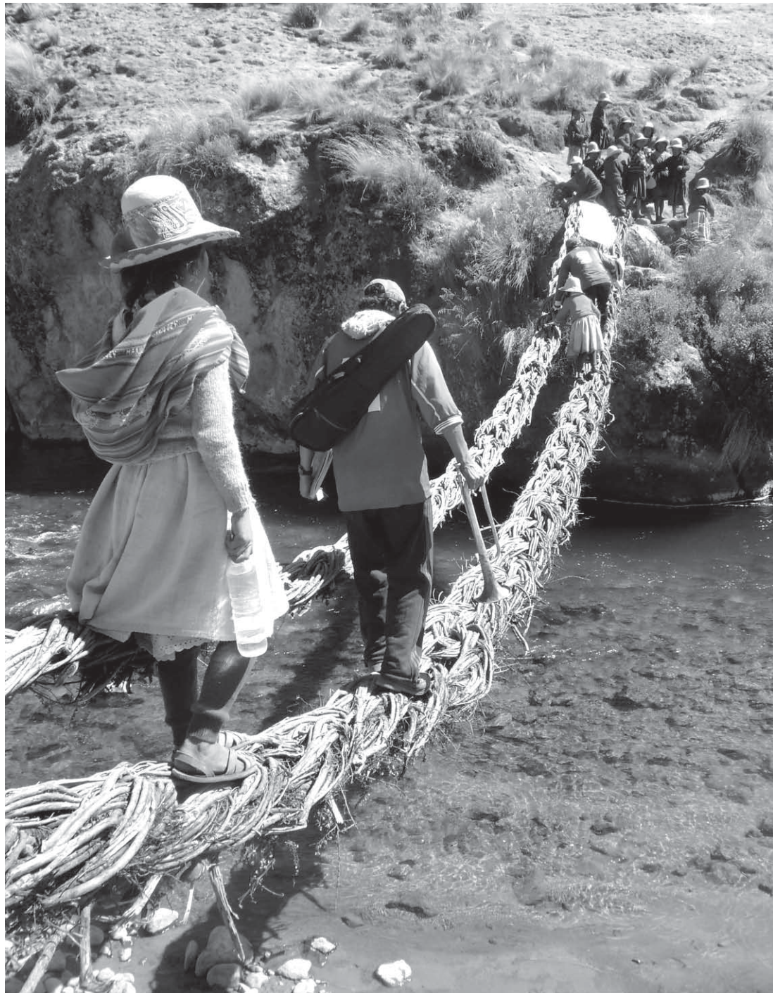
Before the Continental Crossings project, people living in and around Yavina, Peru, had to use this makeshift walkway—two braids of twigs and reeds.
