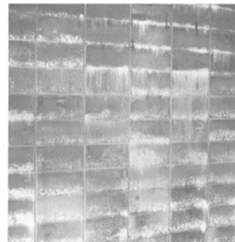
Fig. 1. Photo of masonry wall.
